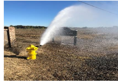
Distribution System Flushing
